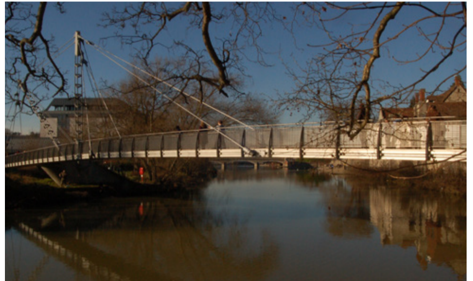
Pedestrian bridge to the east of the site links to the town centre.
