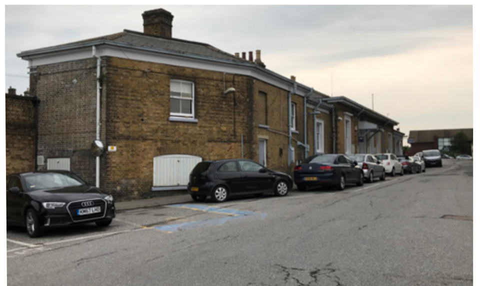
Frontage to Maidstone West Station - opportunities for improvement to public realm and vehicular circulation
