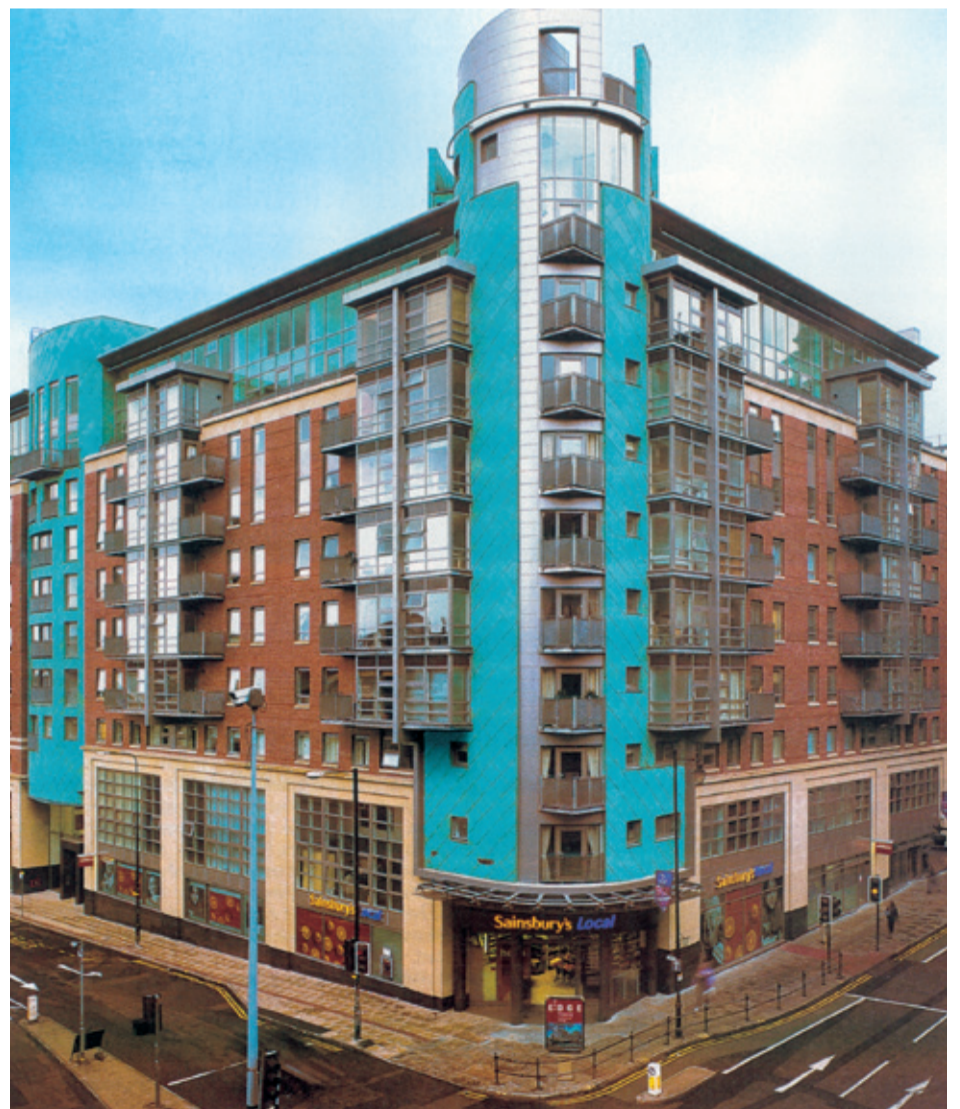
Apartments over supermarket within a landmark building
